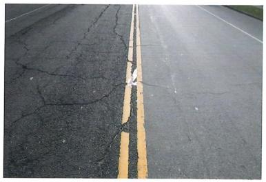
This photo shows a roadway divided by two counties. The one on the left went the Mill & Fill route while the one on the right chose to add a micro-surfacing treatment to the mix. The difference between the two surfaces four years later are dramatic!
